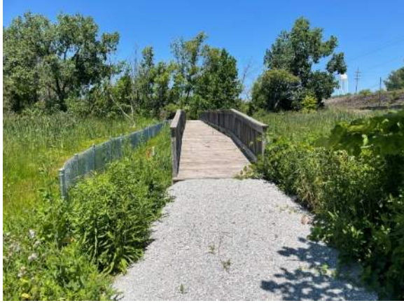
Boardwalk and native plantings in Park 565/Indian Ridge Marsh
