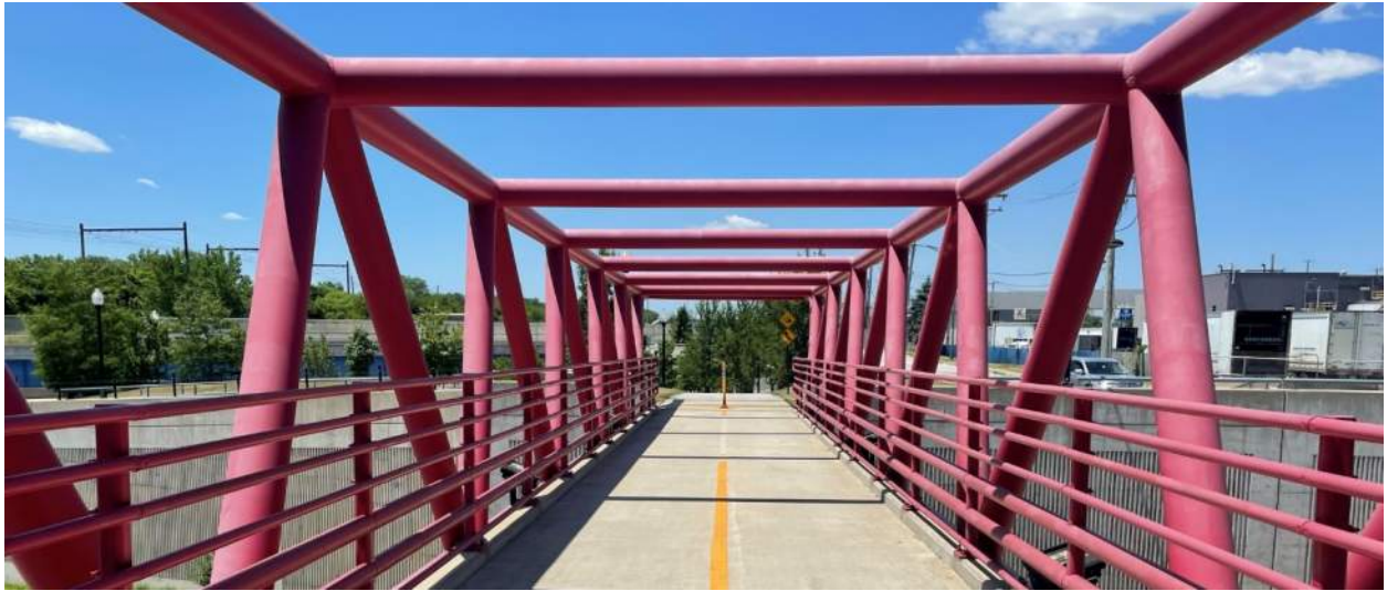
130th Street Bicycle and Pedestrian Bridge
