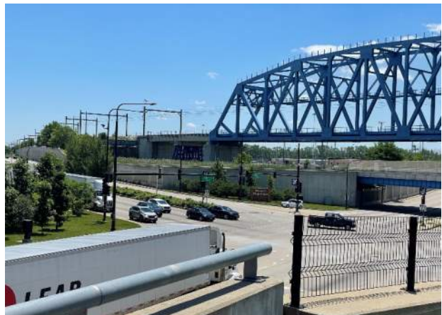
130th Street Railroad Bridge over Torrence Avenue
