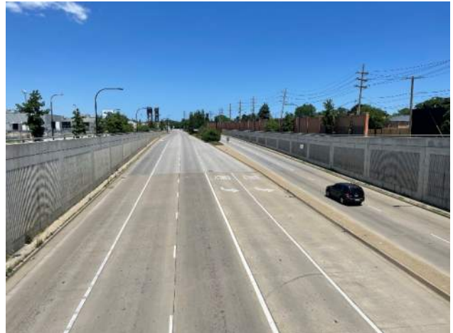
Torrence Avenue at 130th Street, LTS 4.
